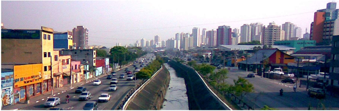
[Fig.4] Ipiranga stream inserted in the urban context. margins contained by trapezoidal section in concrete and floodplains occupied by Ricardo Jafet Avenue
